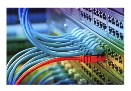
Structure cabling is the design and installation of Cabling to connect the various telecommunication devices and equipment. The structure cabling design and installation is governed by set up standard that specify for the offices, commercial buildings and Data Centres for data and voice communication using various kinds of cables.
